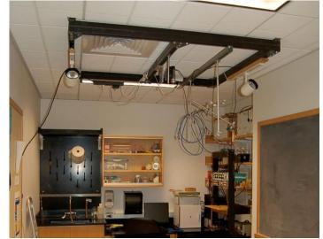
*Figure 7.* Metal framing support system suspended from the ceiling in a recording area of an electrophysiology laboratory. In this example, lights, a commutator, and a video camera are securely attached to the system. (Hamilton College).
